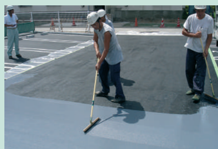
② Coating 1st Coat using Universal Broom (Roller Application also an option)
