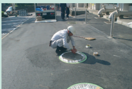
① Cleaning and Masking of existing Road Surface
