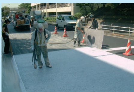
② Spraying Slip-resistance Aggregate
