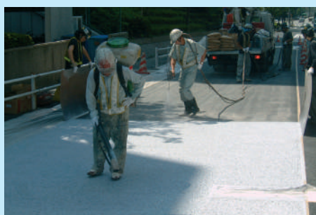
① Spraying 1st Coat with specialized Sprayer
